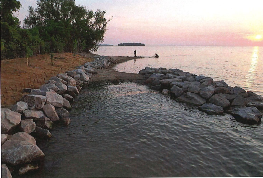
Shoreline stabilization immediately following construction.
